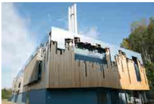
Chaufferie biomasse Wacken
